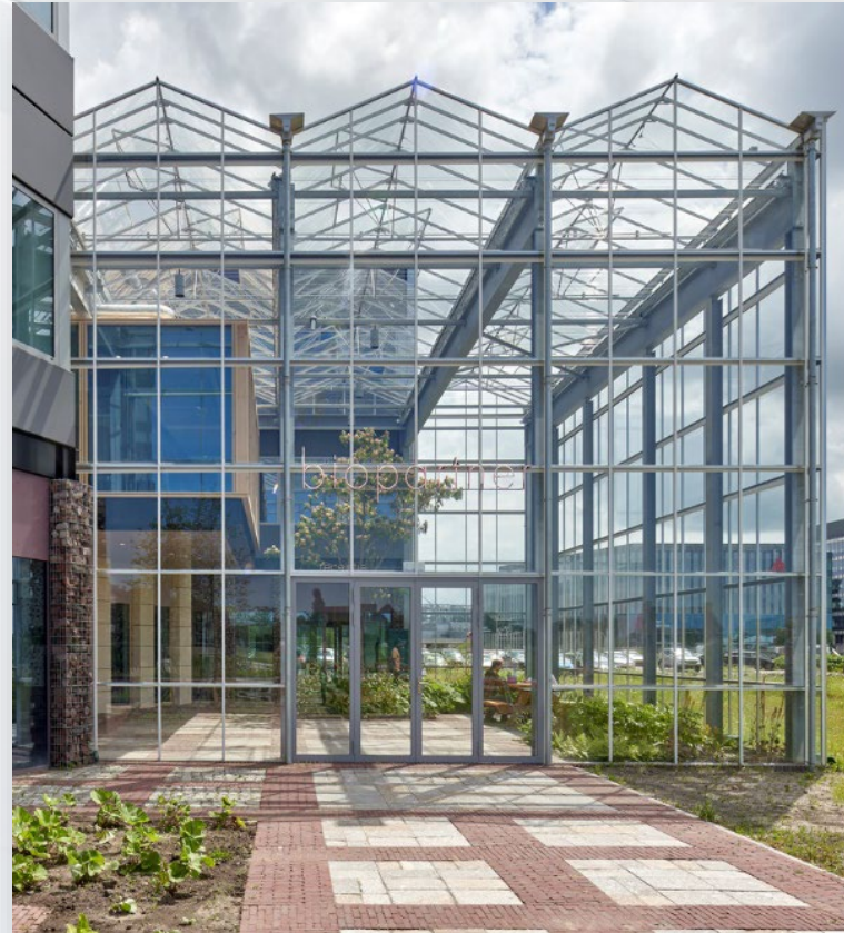
Laboratory: Reuse of 165 t of galvanized steel saves 218 t of CO2
