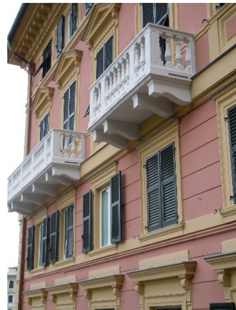
Hot dip galvanized steel reinforced concrete support beams for the balconies of an elegant apartment in Genoa. Galvanized steel reinforcement was chosen to best preserve the support beams of the balconies over time, in particular to protect them from smog, rain, frost and humidity. (Images courtesy of Prefabbricati Torti di Pietro e Lino Torti snc)
