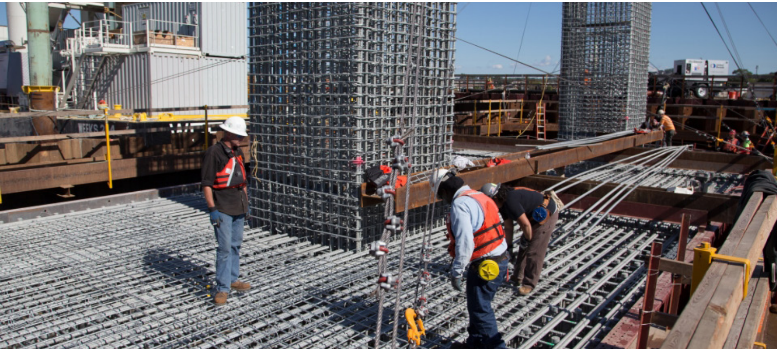
Over 27,000 tonnes of galvanized steel reinforcement ensures the long-term durability of the main span towers, approach span piers, abutments and road deck panels of the Mario M. Cuomo Bridge. (Image courtesy of New York State Thruway Authority)
