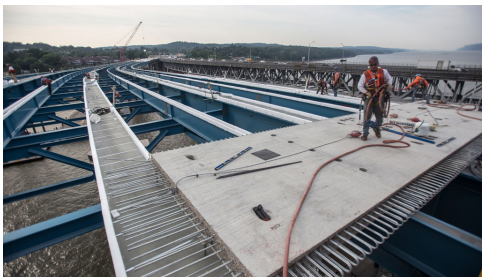
The bridge deck of the Mario M. Cuomo Bridge comprises nearly 6000 precast panels, each 3.66m long and 6.7-13.7m wide, for the approach spans and 963 main span deck panels. The panels are joined by pouring concrete around the protruding galvanized steel reinforcement.
