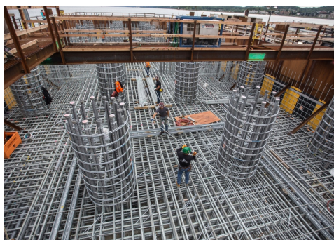
Prior to selecting galvanized reinforcing steel for the Mario M. Cuomo Bridge, the New York Thruway Authority developed a Corrosion Protection Plan to identify exposure, degradation mechanisms, design and construction strategies, and life-cycle costs.
