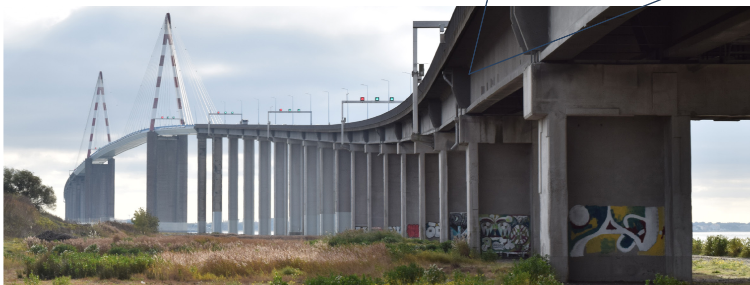
The Saint-Nazaire Bridge was built in the 1970s and is still the longest bridge in France. The majority of its concrete reinforcement was not protected against corrosion and this has led to an extensive programme of maintenance and repairs. Around 63 tonnes of galvanized steel reinforcement was used in very specific locations - the flanges of the T-beam ends and the connection slabs cast in situ at the height of the flanges (pictured above). No repairs have been necessary in the specific locations where the galvanized reinforcement was used.
